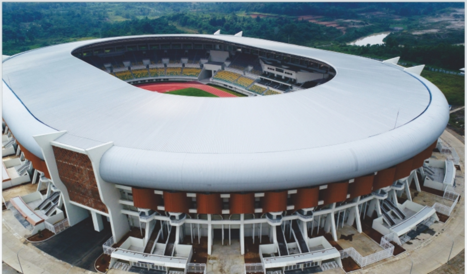
BANTEN INTERNATIONAL STADIUM
